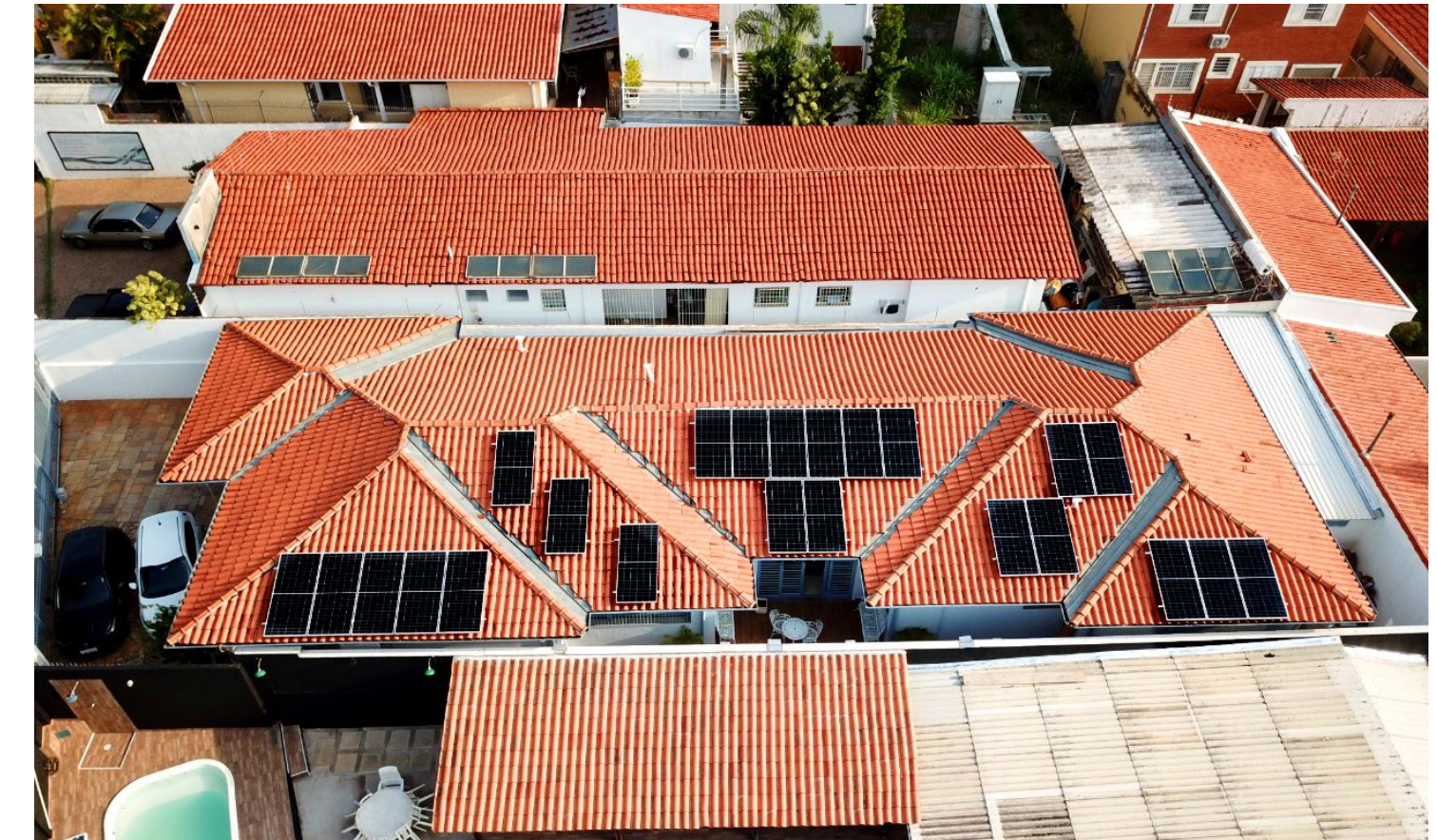
In 2020, DEIF's office in Brazil was fitted with PV solar cells.
